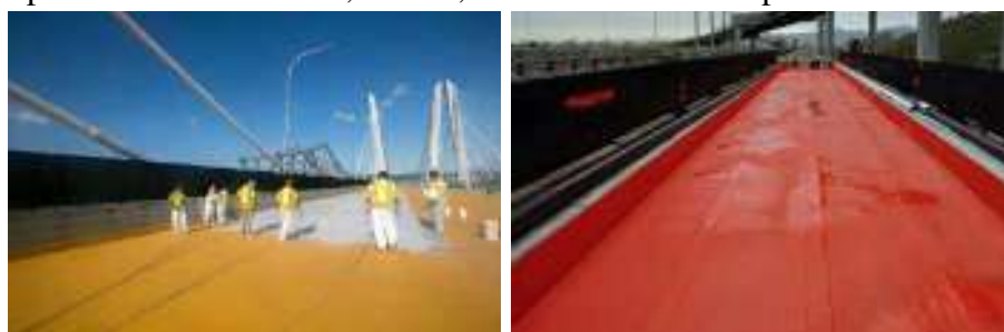
Fig. 5. Installation process of applied waterproofing membranes
