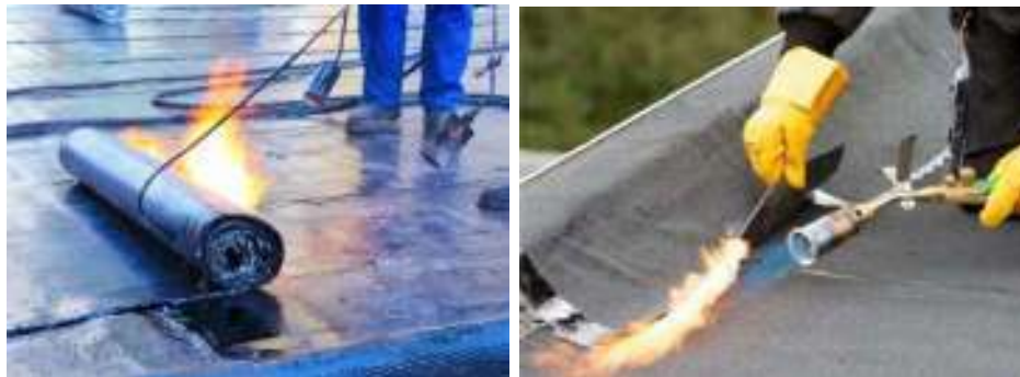
Fig. 4. The installation process of adhesive waterproofing materials
