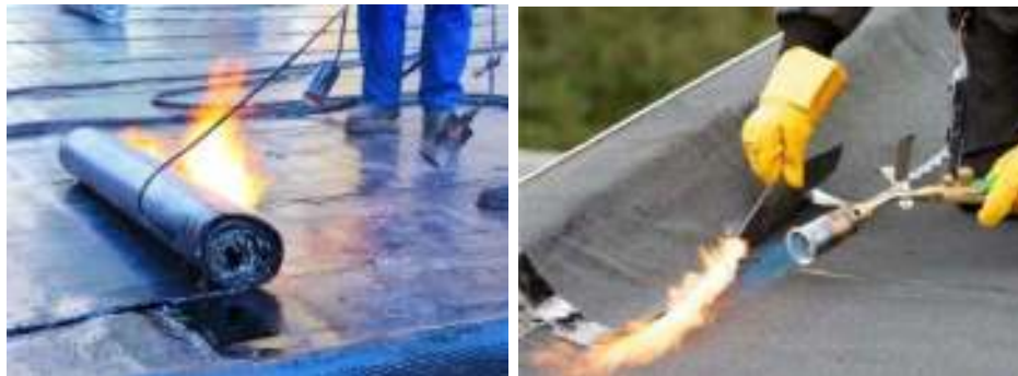
Fig. 4. The installation process of adhesive waterproofing materials
