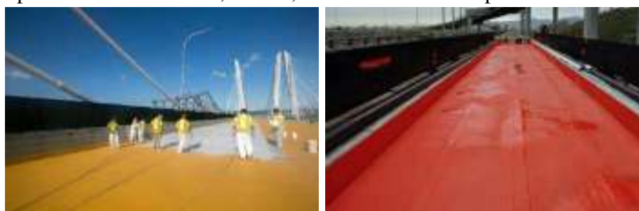
Fig. 5. Installation process of applied waterproofing membranes
